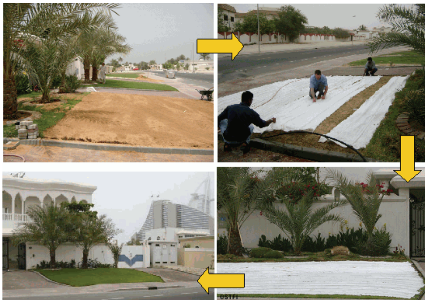
Figure 4: Reference object - installation of irrigation mat in Dubai
